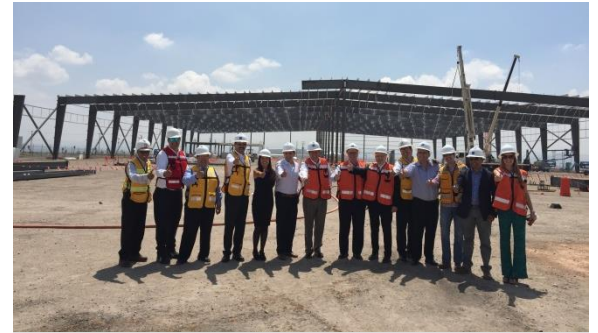
Groundbreaking ceremony, San Luis Potosí, Mexico
